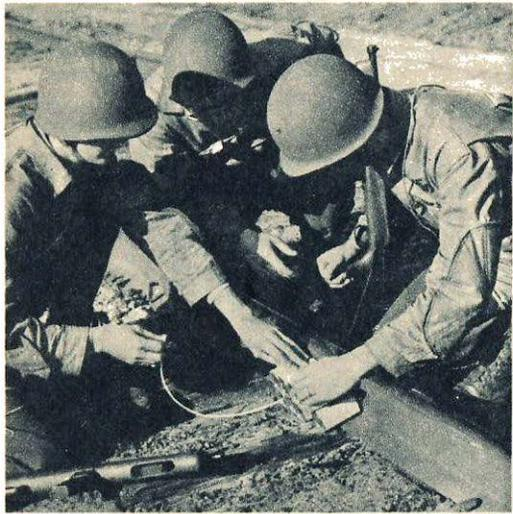
*DEMOLITION is one of the most important phases of training. This group is planting a charge of TNT to blow up railroad tracks. Detonation is shown in picture at right.*
